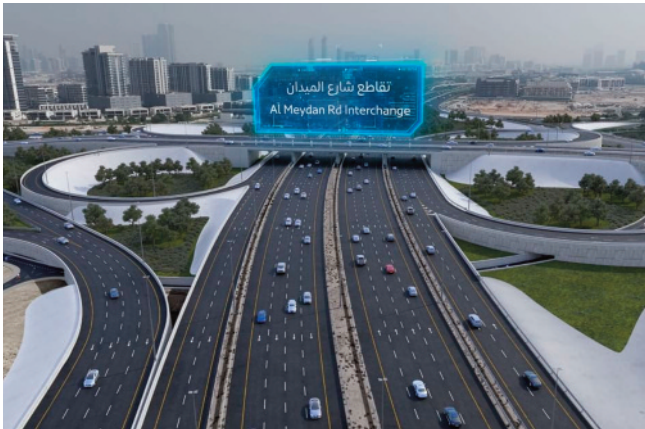
The RTA project includes a direct connection between Al Marabea' Street and Sheikh Mohammed bin Zayed Road, with three lanes in each direction and a combined capacity of 7,800 vehicles per hour —WAM
