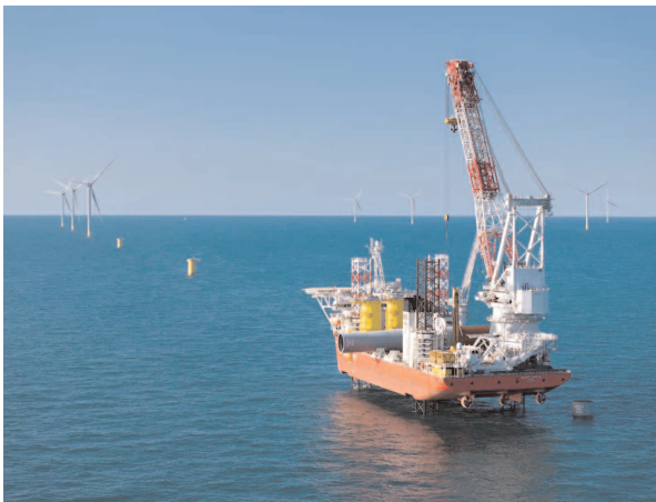
The foundation installation was delivered by Seaway7, with East Anglia THREE the first foundation installation campaign completed by its jack-up vessel, Seaway Ventus
