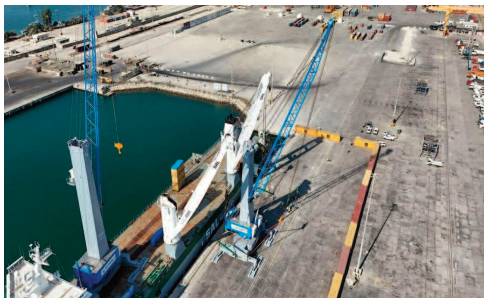
The crane deliveries represent an important milestone under DP World's 30-year concession agreement to develop and operate the Port of Tartous
