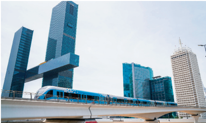
Dubai Metro accounted for the largest share of total ridership during the first half of the year at 39.2 percent, carrying around 136.5 million passengers on the Red and Green lines: Al Tayer
