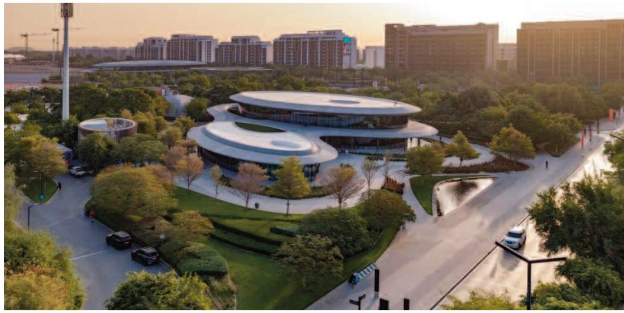
The financing has been linked to Arada's Sustainability Performance Targets (SPTs), which will be measured on an annual basis through the tenure of the facility
