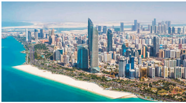
Amid an increasingly complex global environment, Abu Dhabi continues to ensure fluid trade movement, reduce friction across supply chains, and operate with consistency
