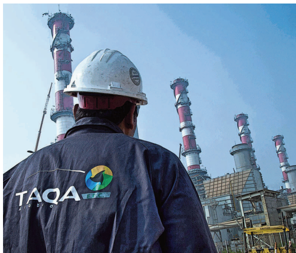
The AI Dhafra OCGT project in the UAE, to be built by Taqa and Emirates Water and Electricity Company, will deliver up to 1GW of baseload power daily, generated from renewable energy
