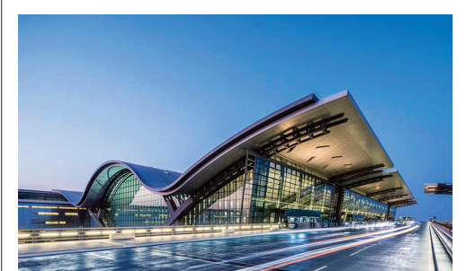
Hamad International Airport's new concourses integrate seamlessly into the existing terminal, introducing cutting-edge technology and enhanced facilities to meet growing passenger demand
