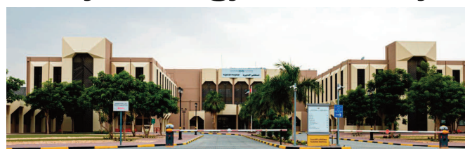
Fujairah Hospital becomes the first government hospital in the UAE to receive LEED Gold Certification from USGBC — WAM
