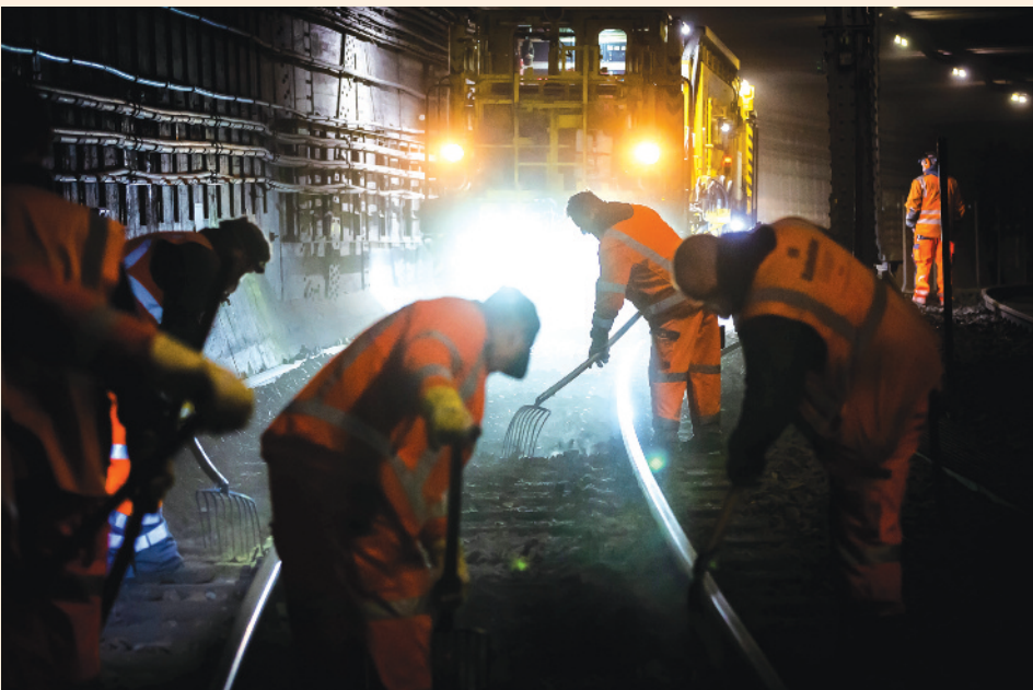
Workers profile the track bed behind a tamping machine that compacts the ballast during a site inspection of the north-south tunnel of the Berlin S-Bahn between the Oranienburger Strasse and Friedrichstrasse S-Bahn stations on Friday —DPA
